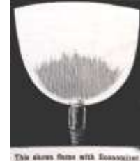
Sold in 1896 by FS&Co as the 'Sun' burner. Left without- right with 'Economizer'.
