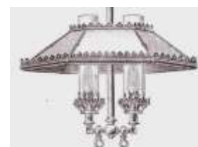
1886. Made by Julius Pintsch, Berlin. The first gas mantle burner of Dr. Auer von Welsbach.
